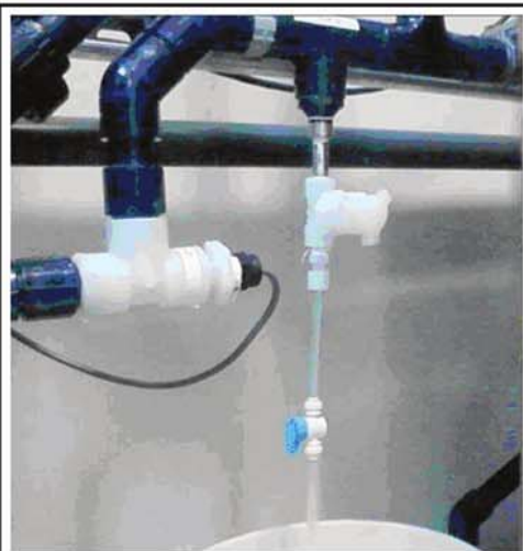
Figure 4. Second sampling valve added at the end of an existing sample line.
