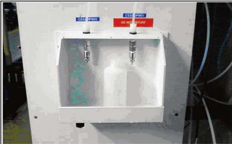
Figure 8. A sample box not large enough to accommodate a sample bottle without touching the bottle neck to the end of the port.
